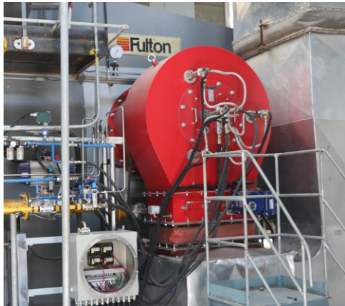
天津旻昊中安信科技项目3台25 吨超低氮30毫克燃烧器改造项目 Anxin Technology Project, in Minwuzhong, Tianjin, 3 sets of 25 tons ultra-low nitrogen 30 mg/Nm3 burner renovation project
